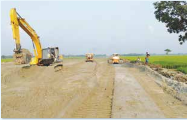
Padma Bridge Rail link Project (Embankment Work)
